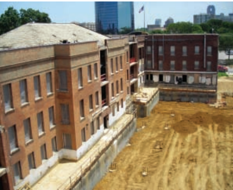
Rear View, 2007 - Good Fulton & Farrell Architects
