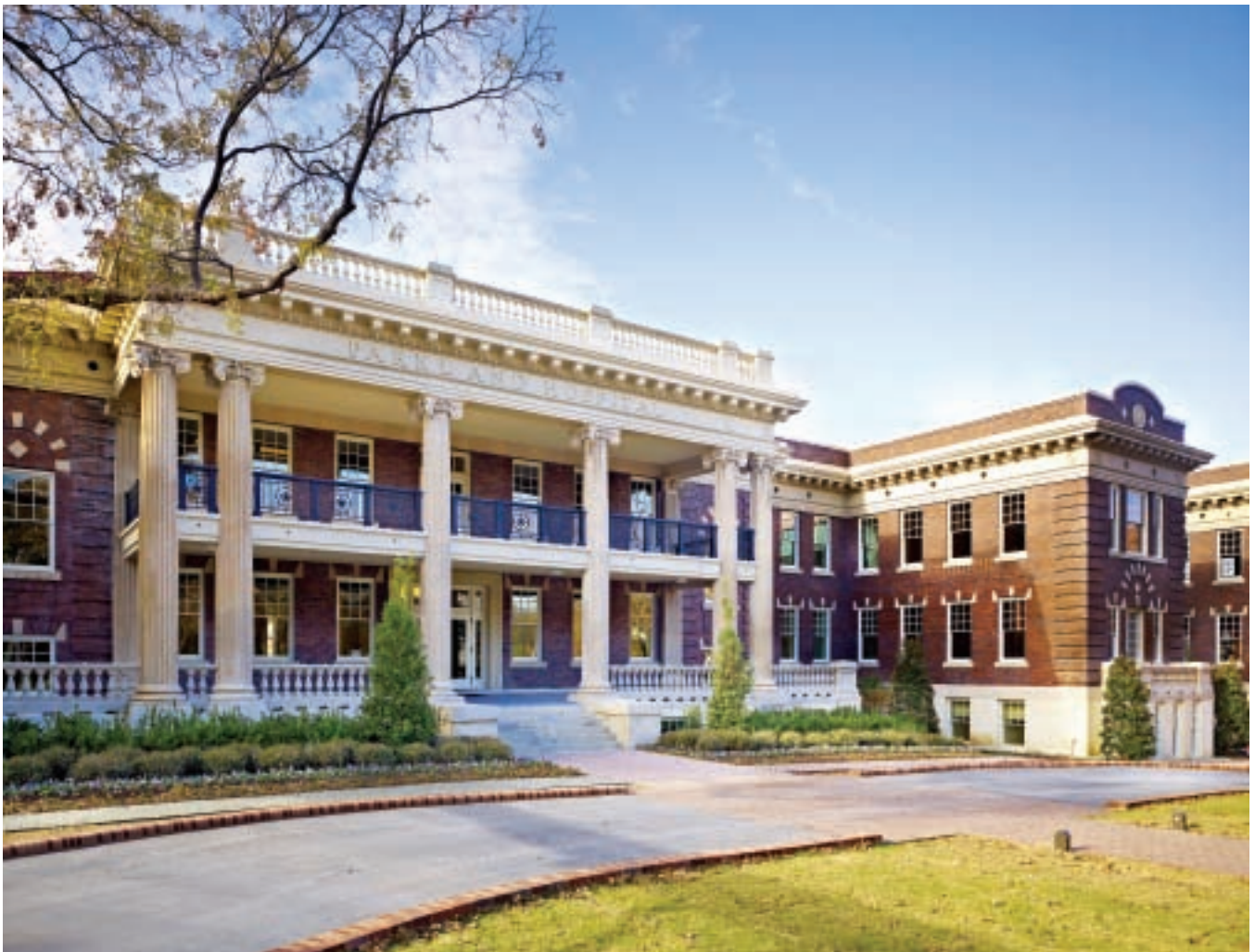
Maple Facade, 2009 - John Davis, DVDesign Group
