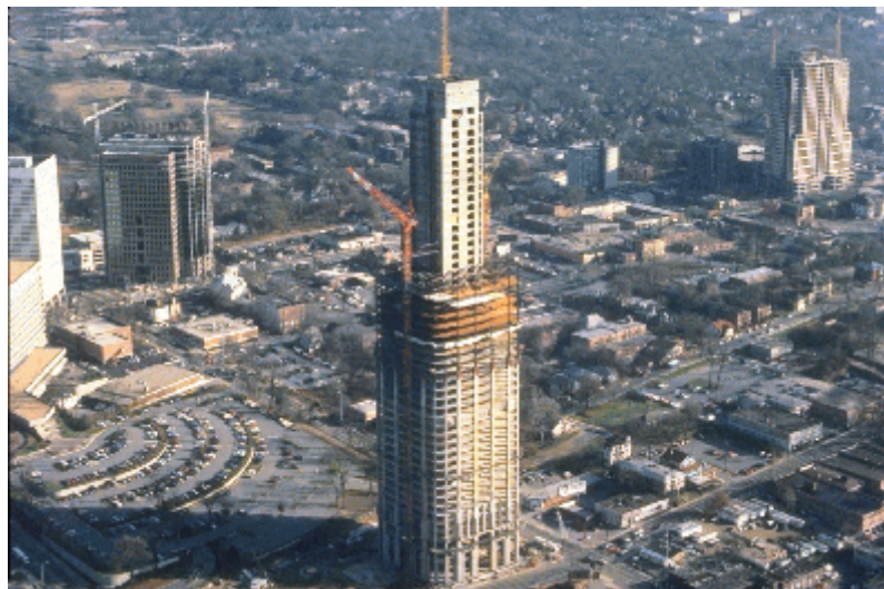
Figure 1 Atlantic Center/IBM Tower Atlanta, Georgia
