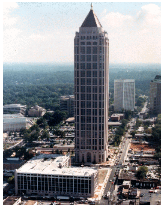
Figure 3 Atlantic Center/IBM Tower Atlanta, Georgia
