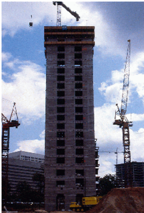
Figure 2 Atlantic Center/IBM Tower Atlanta, Georgia
